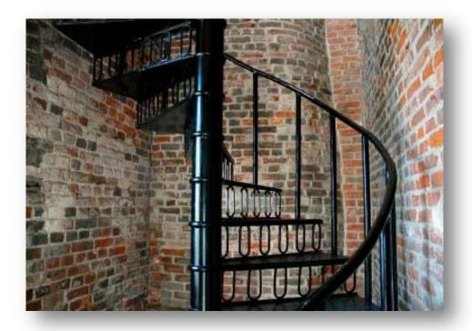
Here is an interesting spiral staircase with an innovative riser that allows the stair to feel open while still performing the function. This is a very simple treatment with the steel complementing the aged brickwork. Purely functional but correct in its application and execution.
